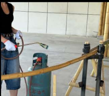
Bend the bamboo to form the door's frame
