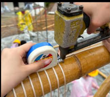
Fixed details: Use a staple gun to drive it in
