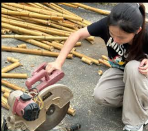
Use a cutter to cut bamboo
