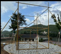
Finish the upper part to form the overall frame
